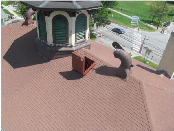
Main roof with new hatch.
